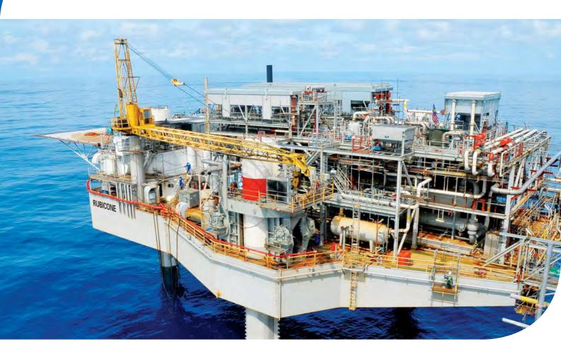
The **Rubicone** is a Malaysian ABS Class Mobile Offshore Production Unit or MOPU, converted in 2011 from a BMC-250 Mat Supported Jack-Up Platform. Equipped with a rack and pinion elevating system powered by Hagglunds motors. Weighing at 5,113 tonnes, it has a daily production capacity of 165 MMscfd of gas, 5,262 BPD of oil and 2,044 BPD of water.
